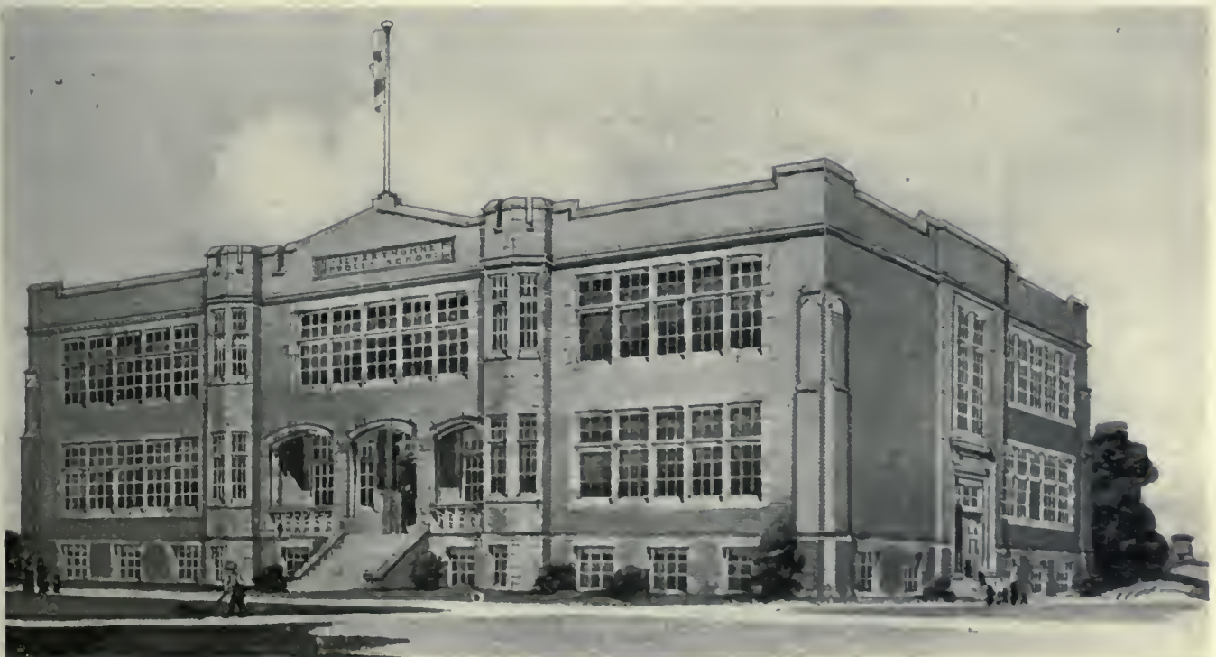
Silverthorne Public School, Mount Dennis now under course of erection.
